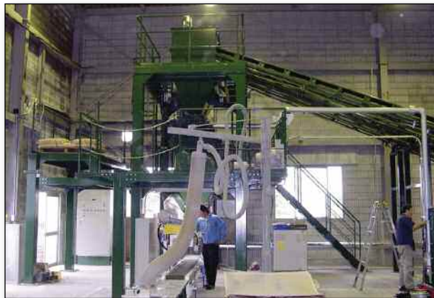
Renewal of the Kumagaya Emcol Plant
