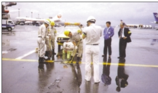
Repairs to roads and runways in Japan with IRR
