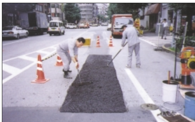
Repairs to roads and runways in Japan with IRR
